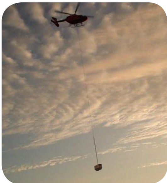
Generator being flown into position
